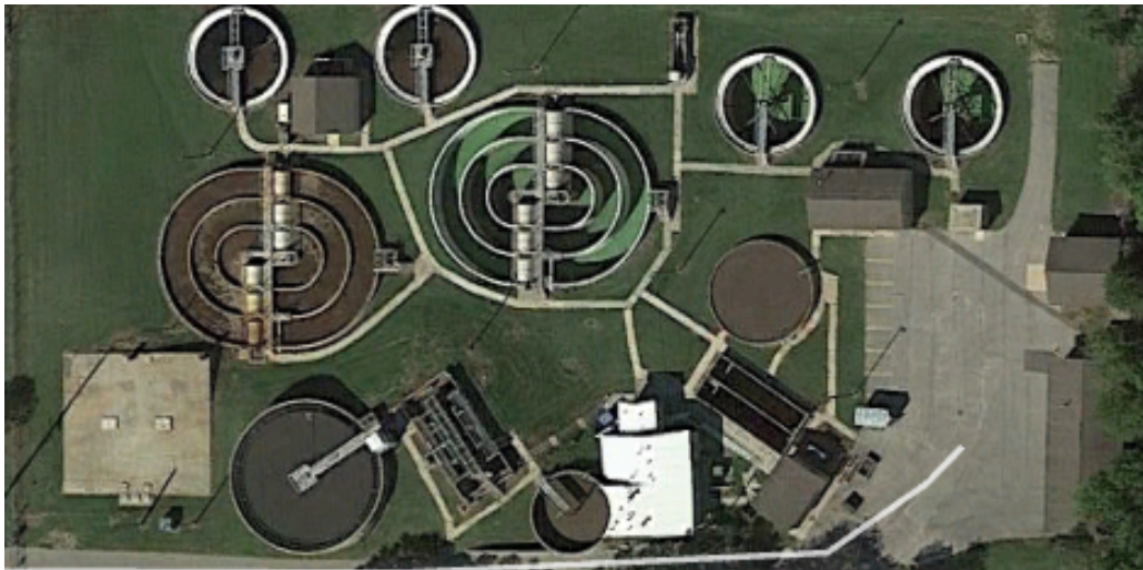
Mechanical Treatment Overview
