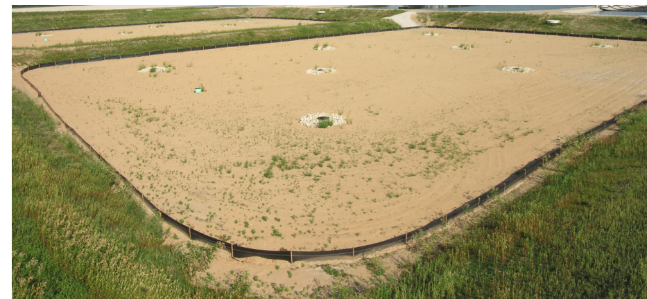
Rapid Infiltration Basin
